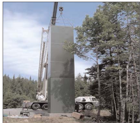
Lime Doser being lowered into position near the river
